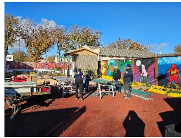
Garden Shed Being Built
